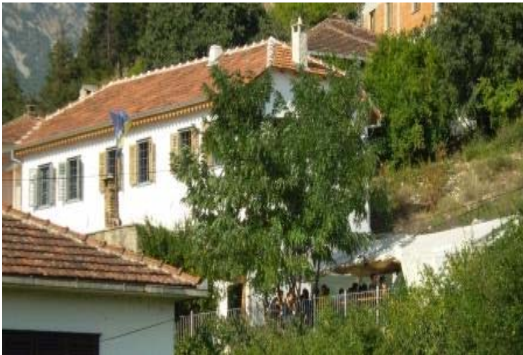
Restored Mehmedbašić endowment house
