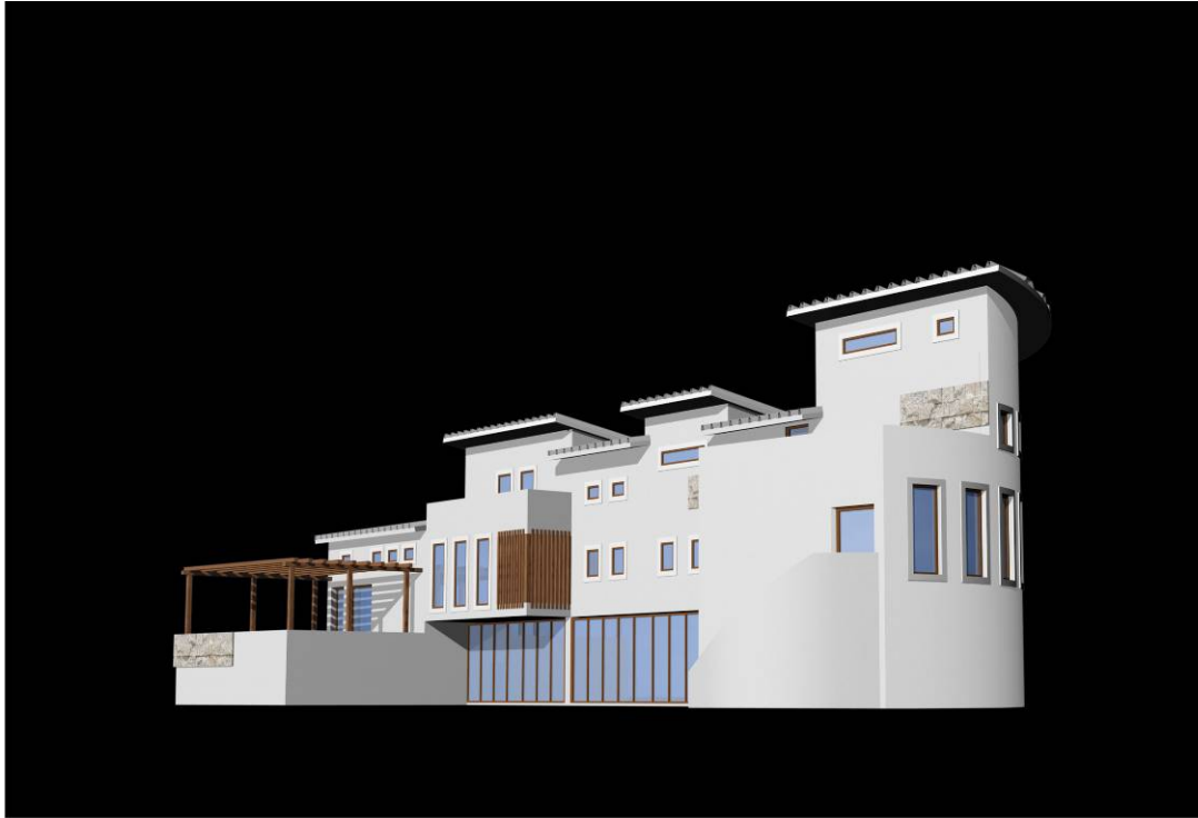
View from the east towards the new building and its inner courtyard
